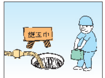
◆ 下水道施工抽廢氣 Circulating & Exchanging Fresh Air in Sewerage.
